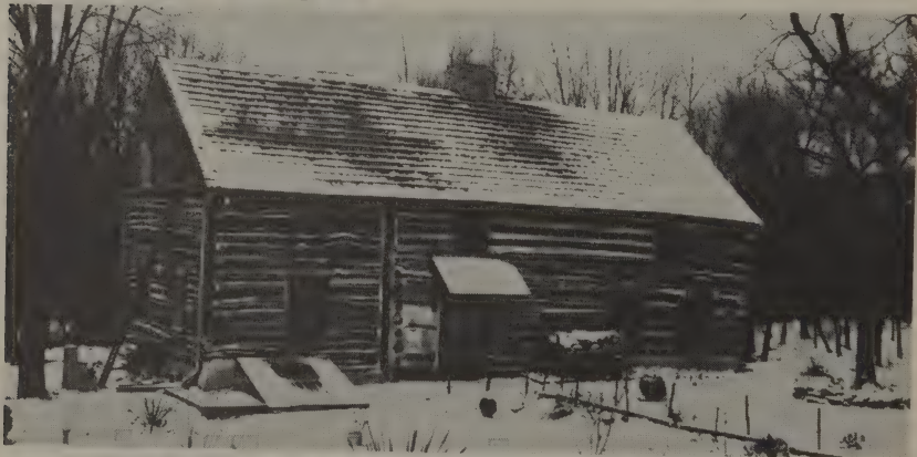
This building, now known as the Shelter House, is a good example of the simple log cabins put up by our German pioneers before the arrival of the Moravian Brethren in Maguntsche. The German settlers reared their chimneys inside and not at the gable-end. The part to the left was added somewhat later.
